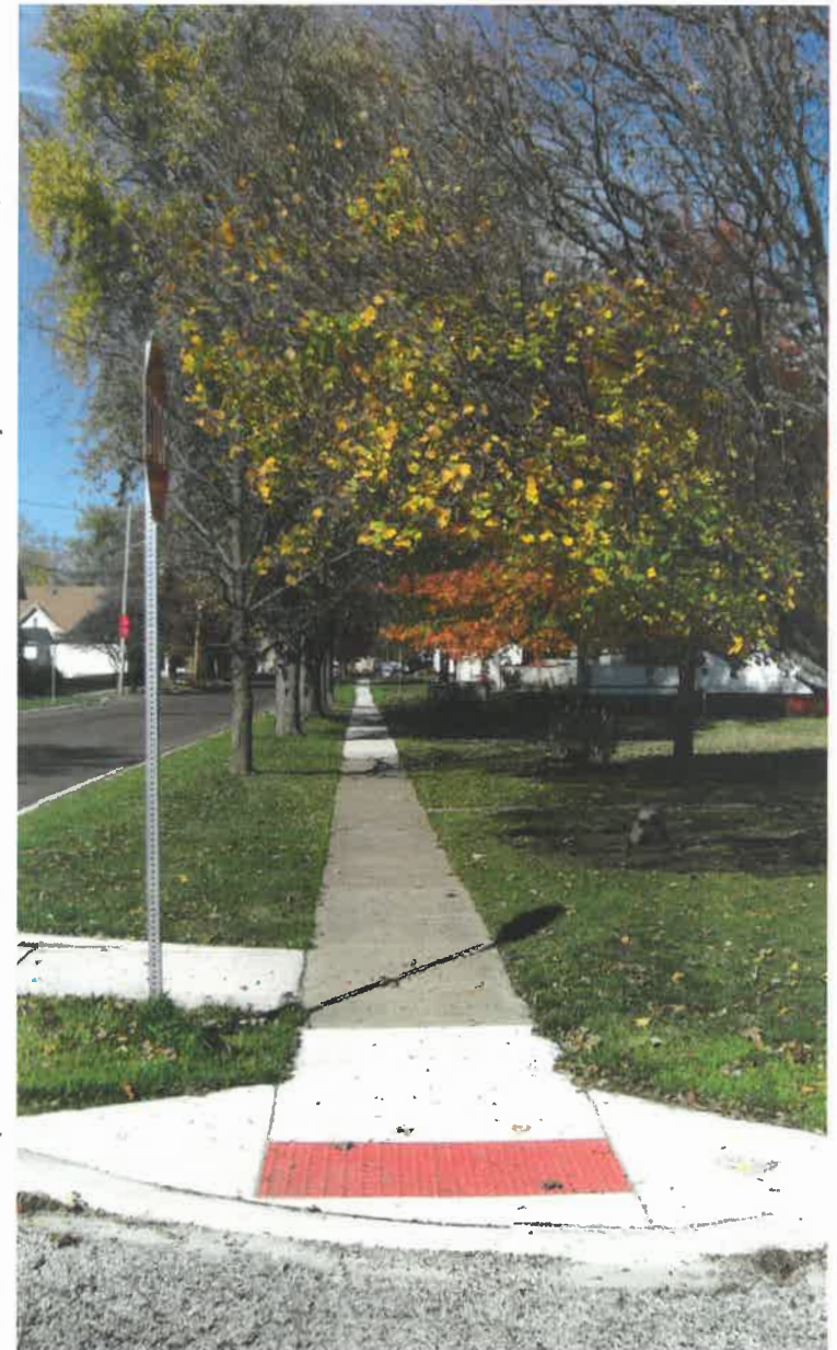
Mackinaw has updated their sidewalks and curb cuts in some areas. The sidewalk shown is located on the east side of County Hwy 6.
